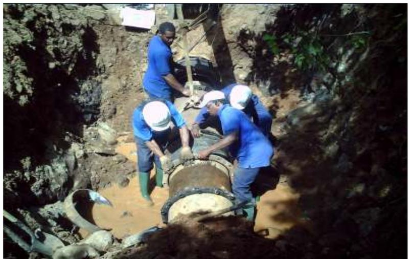
*DOWASCO workers repair a leak on the bulk water pipeline which will be used as the hydropower penstock for the NHP*
