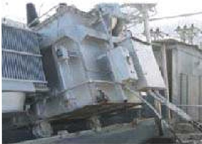
Substation Transformer damaged in Earthquake
